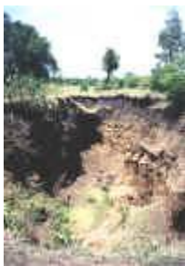
Severe erosion in Nyakach
